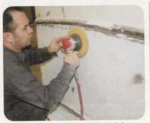
Important Tip: John uses a rotary grinder while the filler is still somewhat plastic to the touch. Other tools that can be used are a "cheese grater" or very coarse sandpaper (40- to 80-grit). Working the surface while it's still curing allows the high areas to be reduced more quickly and with less effort.
