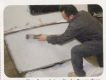
Important Tip: Soon John attacks the surface with a long foam sanding pad, working in an X-pattern to prevent flattening the panel. Some of these long foam sanding pads are supported with metal rods to keep them slightly curved. Remember all exterior surfaces are compound curves (in both directions) from side-to-side and top-to-bottom.
