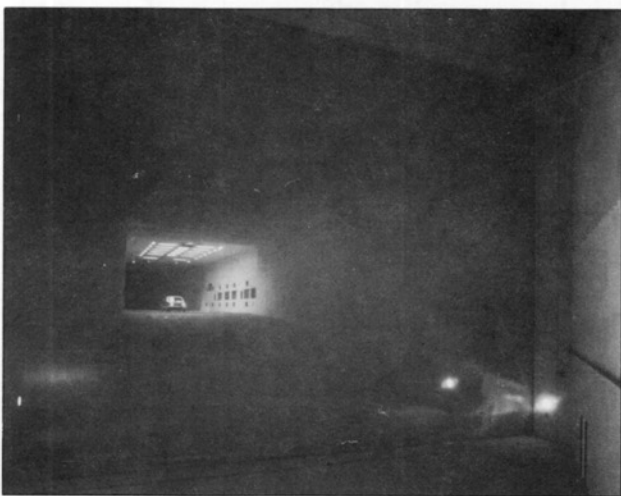
Figure 11 — Flow screen and contraction nozzle from corner 4.
